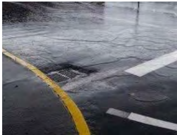
Figure 1: Stormwater draining from a parking lot
